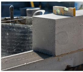
The Thin-Joint method of construction enables a fast, weathertight masonry shell to be built, allowing follow-on trades to start work sooner in a weatherproof environment, whilst retaining the flexibility of on-site construction. Thin-Joint is a recognised Modern Method of Construction and has been fully adopted as the preferred method of wall construction throughout most of northern Europe.
